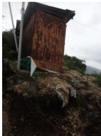
Damage in Bellevue extension camp – Port-au-Prince (Credit: Solidarités international)
