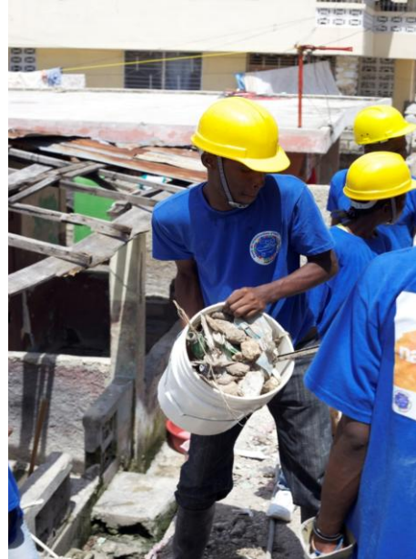
Workers removing debris from inaccessible areas. Photo credit: UNDP
